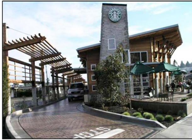
Example of partially enclosed vegetative wall
