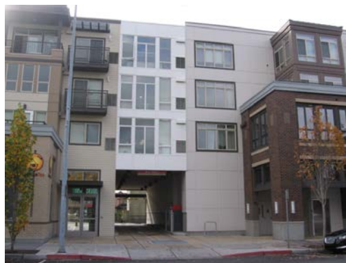
Example of a drive-through within a structure
